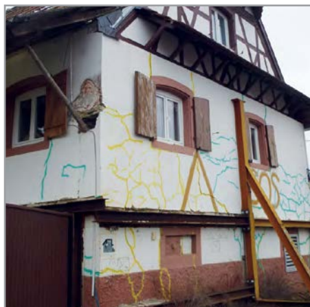
Houses affected by terrain movements in the village of Lochwiller (Alsace- France)
